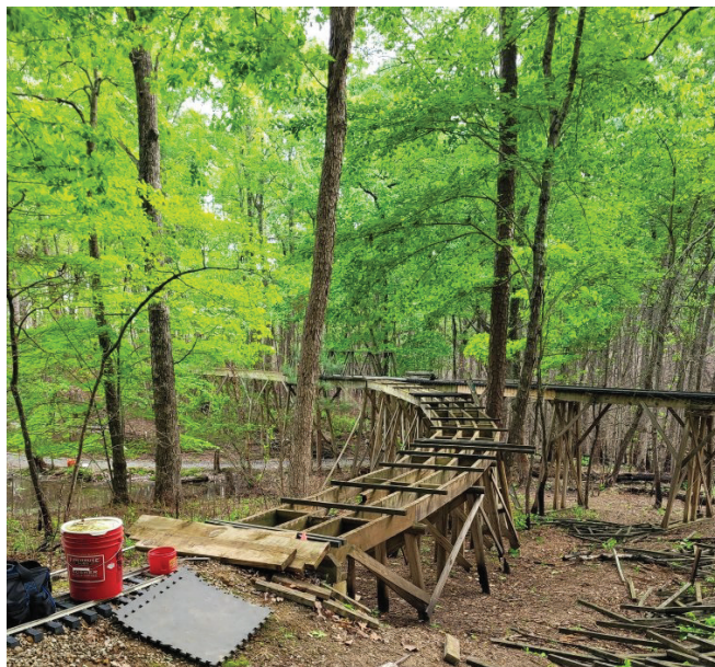
Fig. 9: The curved side of the Kimball Jctn. wye, the side that goes between Deerhead and Sale Creek, has been stripped of ties. Randy Townsend photo.
