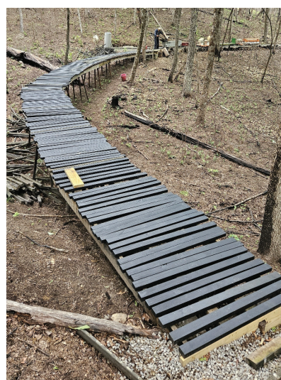
Fig. 5: Ties laid out along the lower Stone Creek trestle prior to being attached to stringers underneath. Glenn Williams photo.
